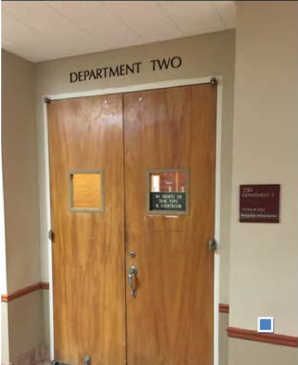
Courtroom 2: Push plate location, exterior. 16" to right of new door. Height 36".
