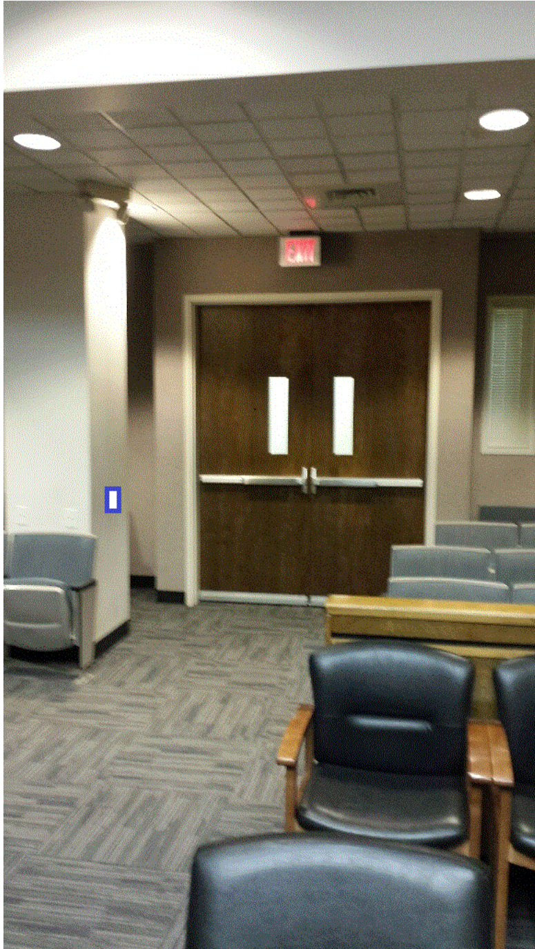
Courtroom 3: Push plate location, interior. Centered on pillar. Height 36"
