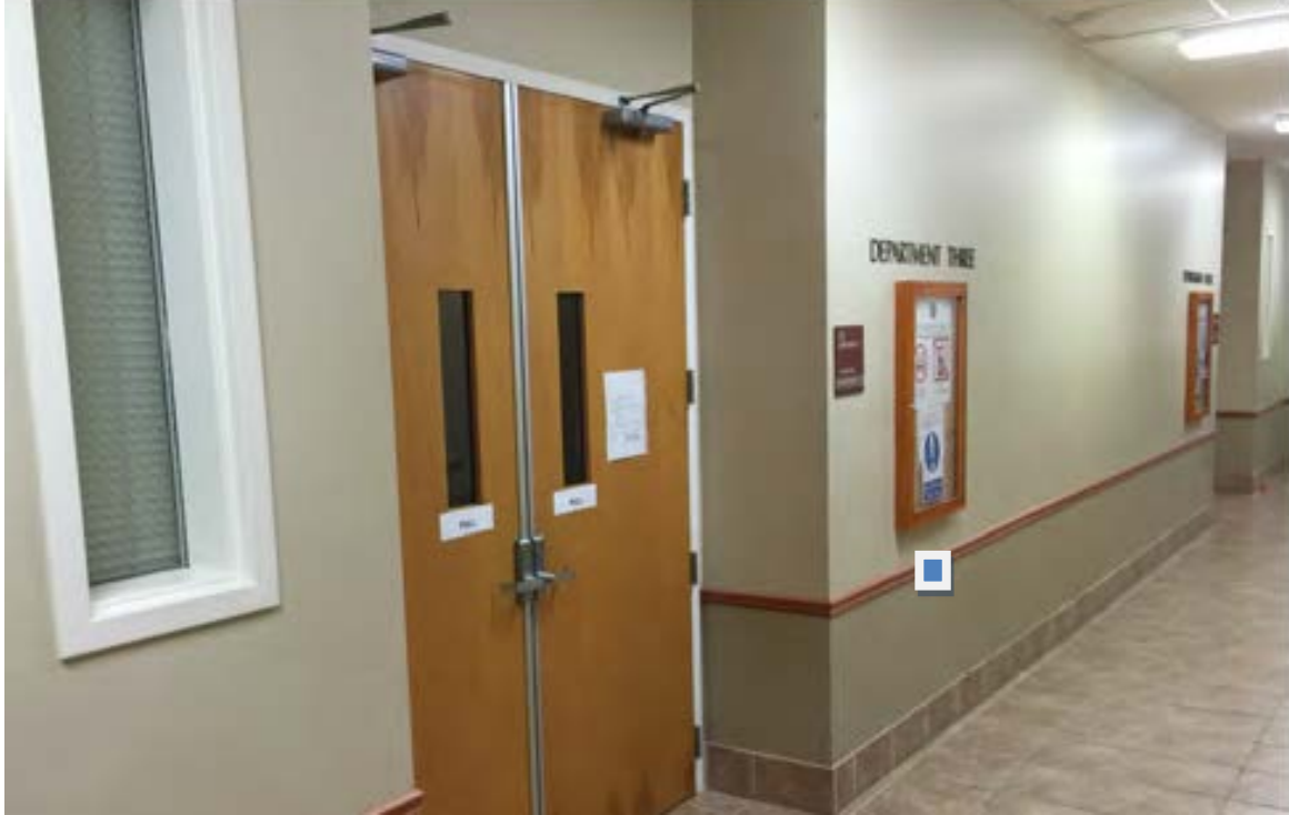
Courtroom 3: Push plate location, exterior. 16" from corner. Height 36".
