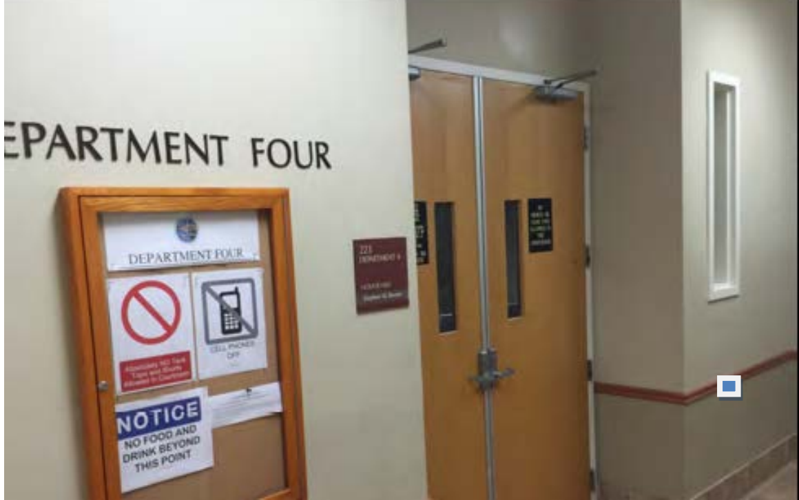
Courtroom 4: Push plate location, exterior. 16" from corner. Height 36".
